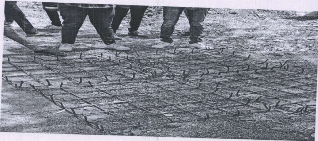
Fig 4: Footing reinforcement
