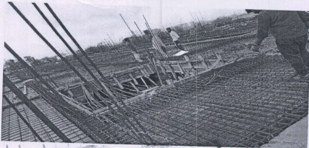
Fig 4: Footing reinforcement
