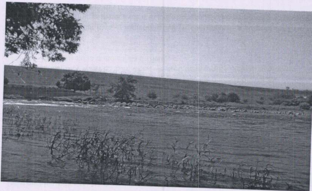
Fig. (c) Chandoli Dam Upstream side
